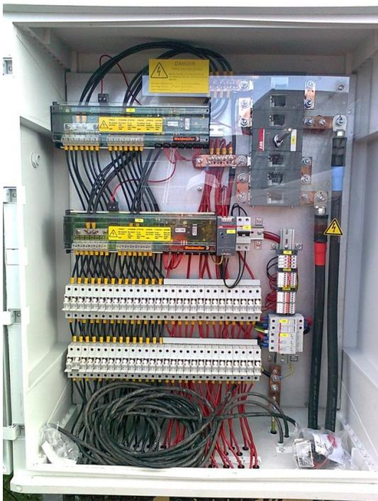
Fig. 6. Experimental junction box and string monitoring
