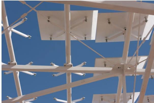
Fig. 3: Mirror facets and supporting system
